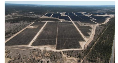
Completed Edenvale Solar Park in Sep. 2023
