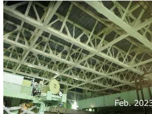
Seismic reinforcement work (Upper part of reactor building)
