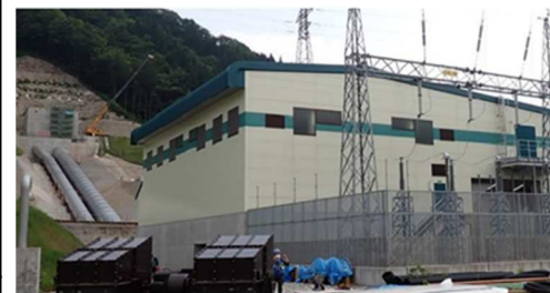
【Tamagawa No.2 Hydroelectric】 Output 14,600kW (Operation Started : Nov.2022)
