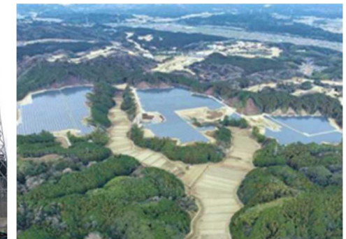
【Power Plant Tsuhaze】 Output 35,000kW (Operation Started : Feb. 2023)
