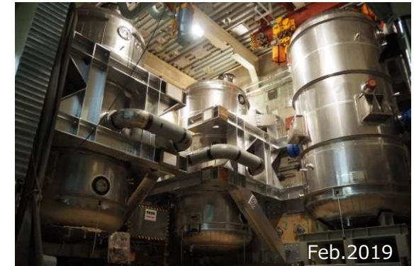
Containment venting system with filter
