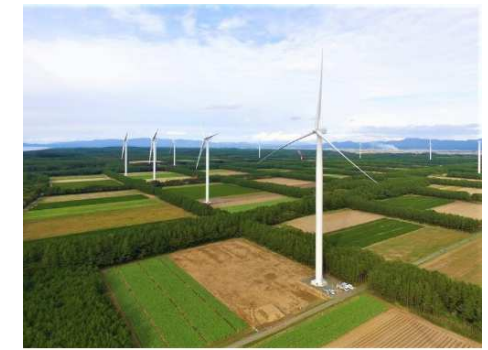
【Windfarm Tsugaru】 Output 121,600kW (Operation Started : Apr.2020)
