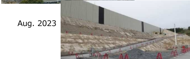
Work for raising the level of the tide embankment
