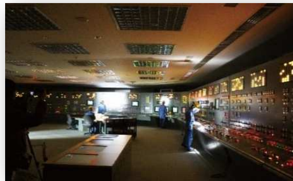
Drill assuming loss of all AC power (Operation simulator training facilities)
