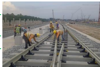
Construction of new lines in Singapore
