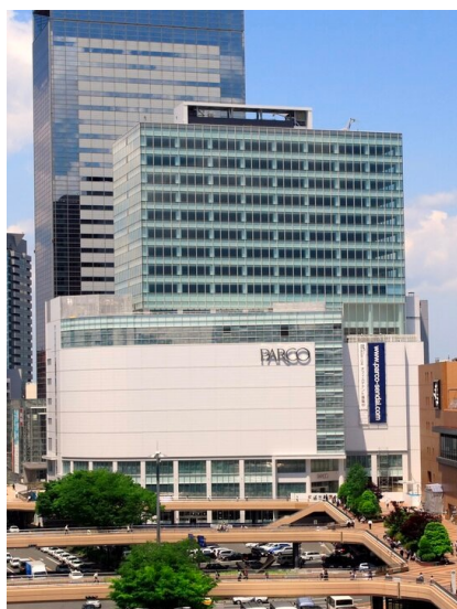
<Sendai Sales Branch入居ビル外観>
