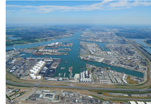
Industrial complex in the Port of Rotterdam
