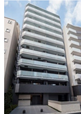
Example of condominium construction
