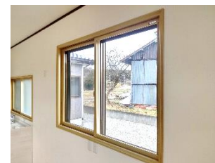
Example of installing double-paned window
