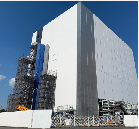
Construction in progress at FJ3
