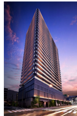
The Parkhouse Kawagoe Tower
