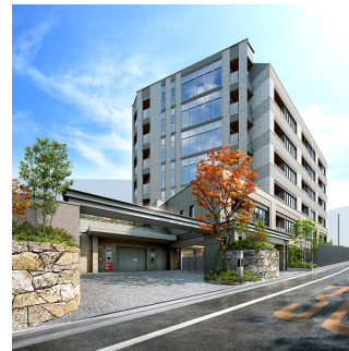
The Parkhouse Takanawa Place
