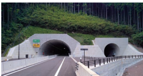
Futaenotoge Tunnel (Aso Block) (Kumamoto Prefecture) 2020
