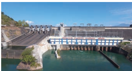
Nam Ngum 1 Hydroelectric Power Plant Expansion (Laos) 2022
