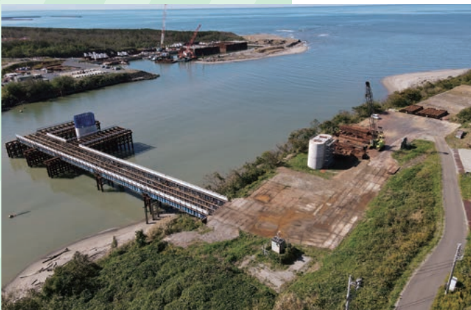
New Nozumi bridge piers.
