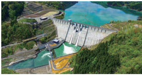
Tsugaru Dam (Aomori Prefecture) 2016
