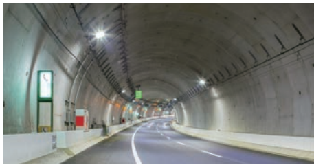
Yokohama Ring Expressway Northwest Route Shield Tunnel (Kanagawa Prefecture) 2019
