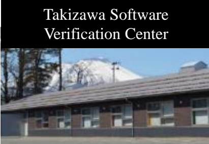
Takizawa Software Verification Center 152-409 Sugo, Takizawa City, Iwate Prefecture Takizawa IPU Innovation Center 2 Laboratory 2-4
