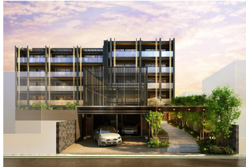
Kawagoe, Saitama Total number of units: 50 Completed and delivered in July 2023
