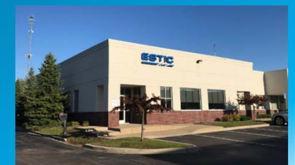
Novi Technical Center
