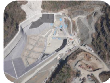
February 2022: Operation New controlled landfill site
