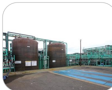
Seki Business Office (water treatment)
