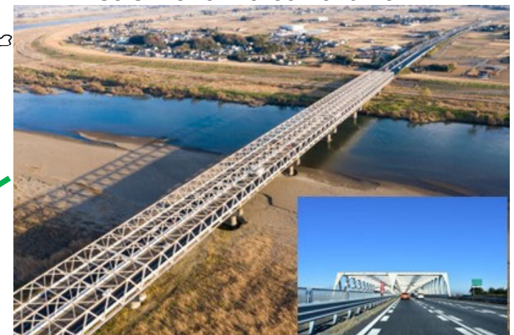
Tohoku Expressway Tone River Bridge seismic reinforcement work
