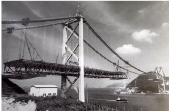
Kanmon Bridge (1,068 m)
