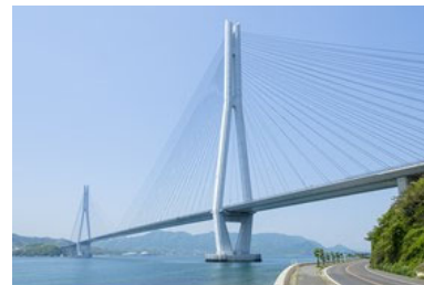
Tataru Bridge (1,480m)
