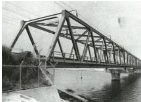
Tokaido Shinkansen Egawa Bridge
