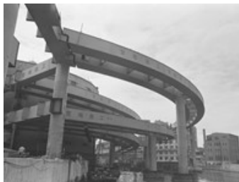
Metropolitan Expressway Edobashi Junction
