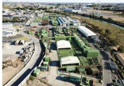
MIYAJI ENGINEERING CO., LTD. Kurihashi Equipment Center
