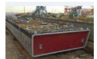
Tokyo Bay Umi-no-Mori Tunnel immersed tube tunnel
