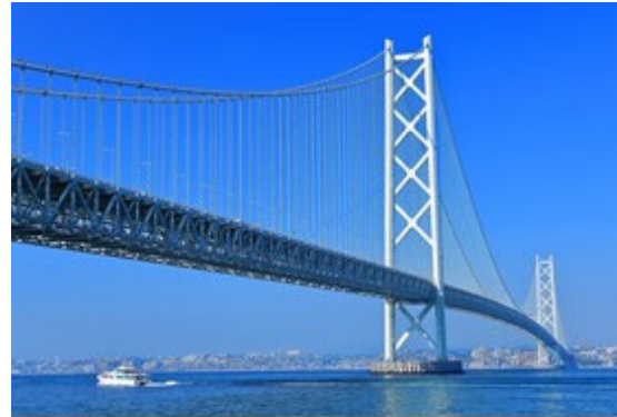
Akashi-Kaikyo Bridge (3,991 m)
