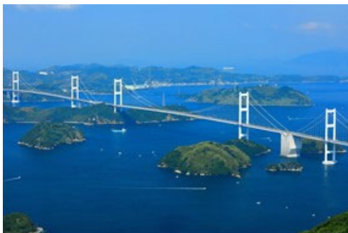
Second Kurushima-Kaikyo Bridge
