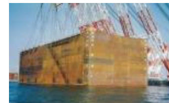
Minami Honmoku steel caisson
