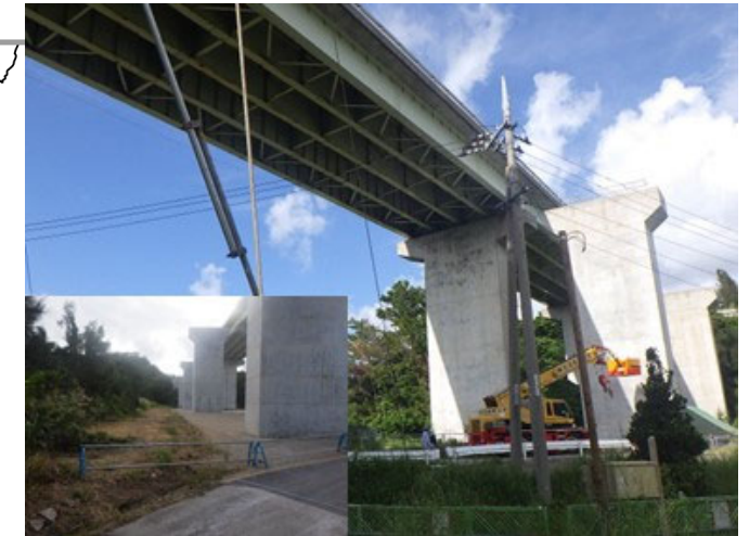
FY2023 Onna BP No. 5 Bridge steel superstructure (outbound) construction, etc.
