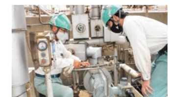
On-site training to enhance inspection capabilities
