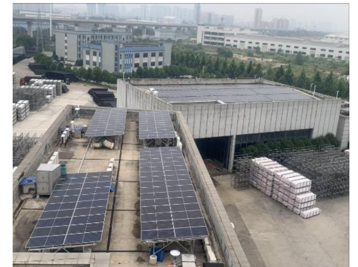
The solar panel installation site
