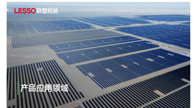
LESSO Solar Power Generation System Installation
