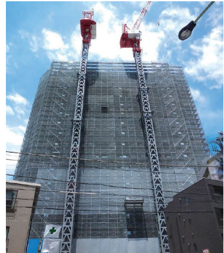
Scaffolding at this 80-meter condominium project begins at the B2 level and has a total height of 90 meters
