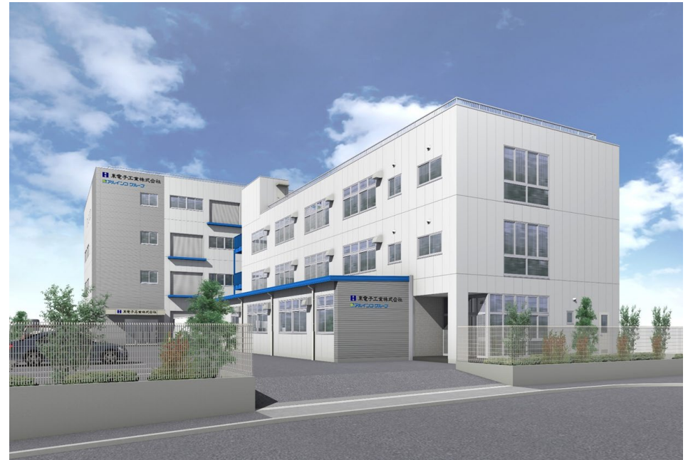
Image of the new plant of HIGASHI ELECTRONICS INDUSTRY CO., LTD.
