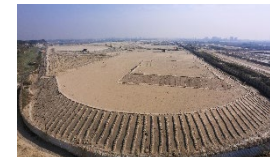
Construction of a depot for railcars in Dhaka
