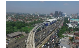
Construction of Mass Rapid Transit, Jakarta
