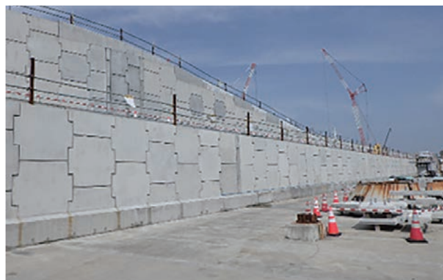
Part of the completed breakwater.
