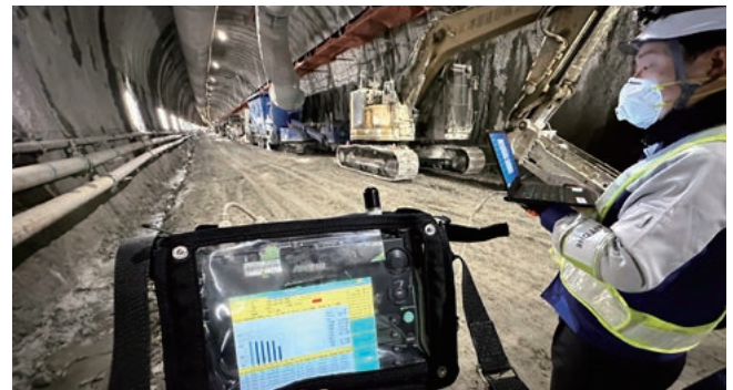
Trial at a tunnel work site.
