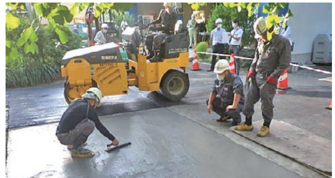
Construction trial using Carbon Pool concrete.
