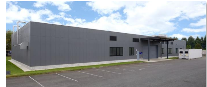
Battery Safety Testing Center
