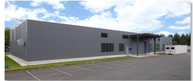
<Battery Safety Testing Center> (within the Utsunomiya Technocomplex)
