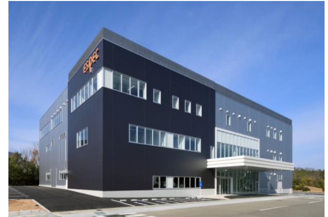
Technology development building
