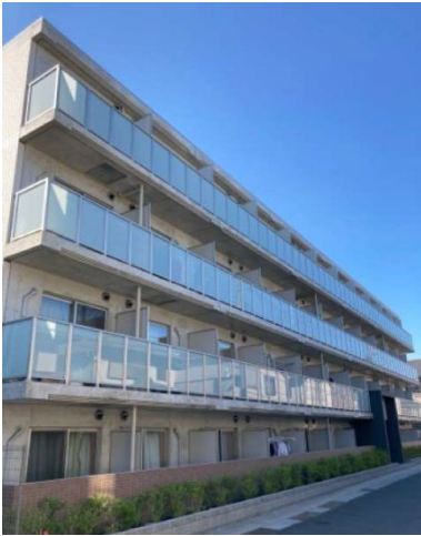
(4) SAMTY Residence Funabashi Kaijin
