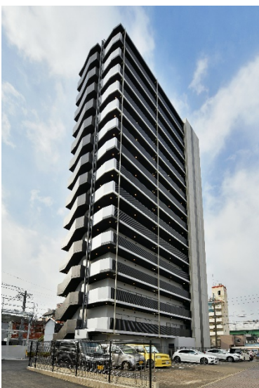
(6) S-RESIDENCE Horita North
