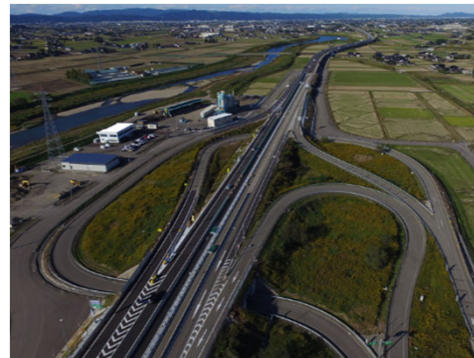
Pavement work on the Tokai-Hokuriku Expressway in Nanto City
