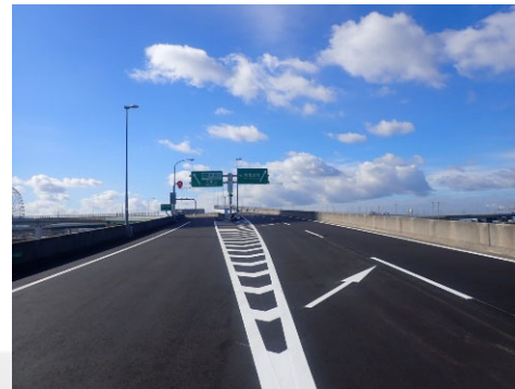
Large-scale pavement repair work (2021-10-Wan)
