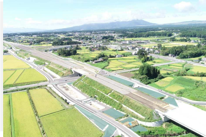
Construction of Shin-Tomei Expressway Gotemba Interchange (Shizuoka Pref.)
