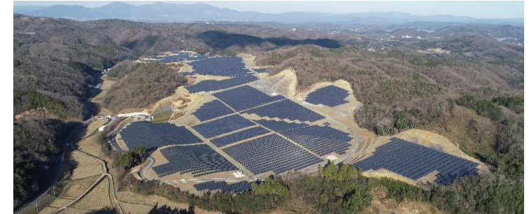
FBIT Misaki Power Plant (Misaki-cho, Kume-gun, Okayama Pref.)
