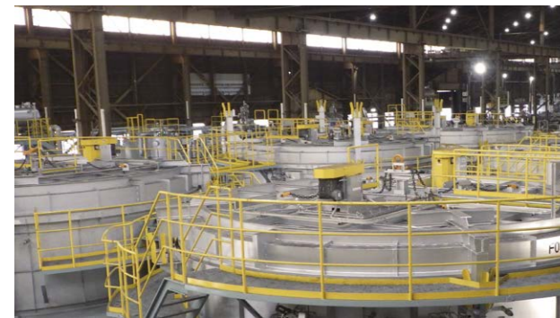
Baking furnace at Plant No. 1, Takuma Division We are carrying out a variety of initiatives to reduce environmental impacts at production sites, for example by saving energy and reducing energy consumption.
