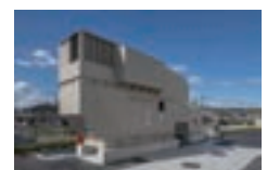
Osaka/Ibaraki Distribution Center No. 5 Emergency generator
