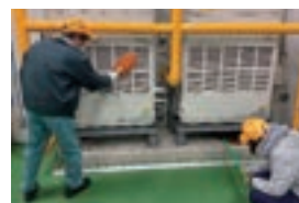
Cleaning under air-conditioning units
