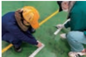
Repairing floor line tapes
