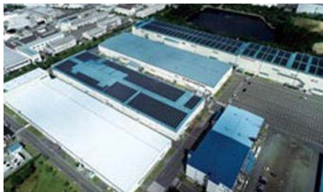
Seishin Works: 728-kW power generation facility
