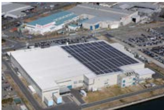
Nagoya Works 1: 750-kW power generation facility
