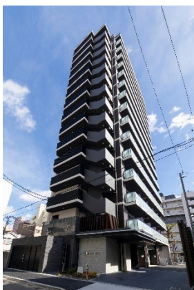
19. S-RESIDENCE 上前津 South
