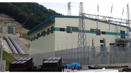
【Tamagawa No.2 Hydroelectric】 Output 14,600kW (Operation Started : Nov.2022)
