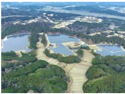
【Power Plant Tsuhaze】 Output 35,000kW (Operation Started : Feb. 2023)
