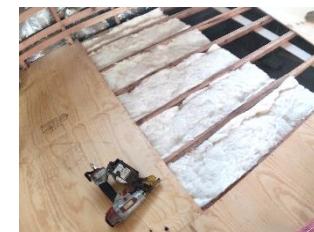
Example of installing insulation
