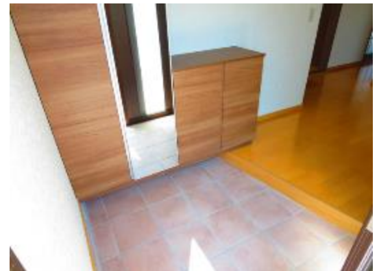
Renovated entrance, by replacing the carpet with flooring, cladding the entrance foyer with new terracotta-style tiles and installing a new shoe closet
