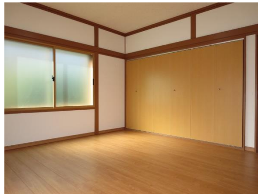
Conversion of two adjoining Japanese rooms into two modern Western rooms, by installing a wall and replacing tatami mats with flooring, at a low cost achieved by using the original sash
