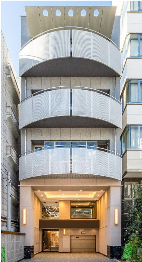
Building exterior Nishi-Shinjuku, Shinjuku-ku 5-story steel-framed reinforced concrete building with one basement floor
