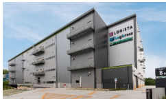
Logista · Logicross Ibaraki Saito (B Building) • Disposed : FY2022
