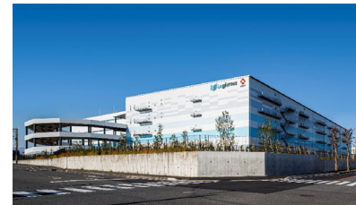
Logicross Sagamihara Completion : Dec. 2023
