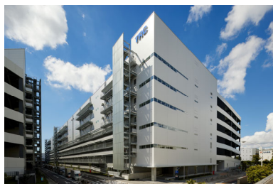
Tokyo Ryutsu Center Distribution A Building
