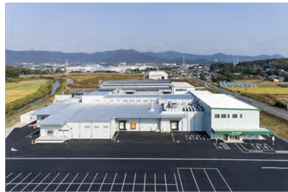
(Working title) New construction of Toyohashi factory of Shokuken Co.,Ltd. (Aichi pref.)
