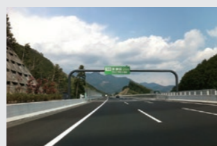
Example of Grandphalt ART use / New Tomei Expressway
