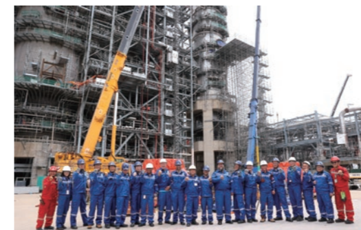
Periodic repair work called Turnaround
