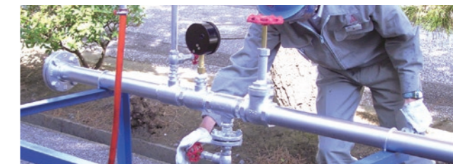
During process safety training
