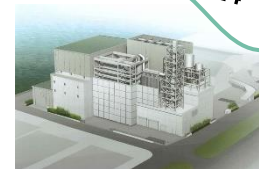
Image of Nishinomiya Energy Plaza
