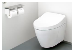
Toilet renewal work (water-saving toilet)
