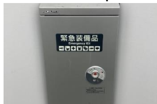
Installation of disaster supplies
