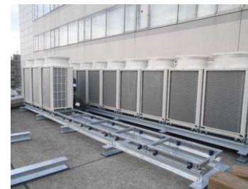
Renewal work to equipment that has energy-saving effects
