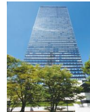
Shinjuku Mitsui Bldg. (Shinjuku-ku, Tokyo)
