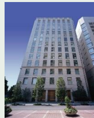
Yodoyabashi Flex Tower
