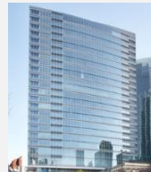
Panasonic Tokyo Shiodome Bldg.
