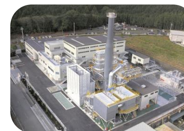
Fujinomiya Business Office (incineration)
