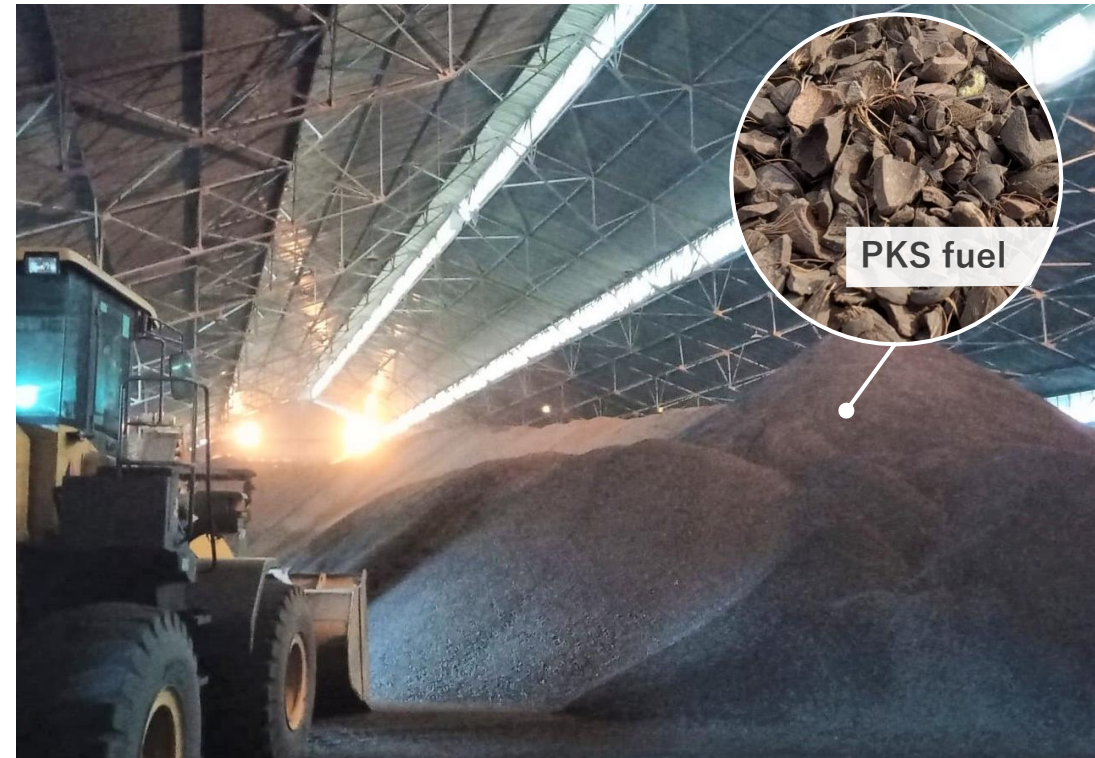
Newly opened stockpile
