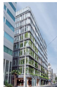
▲ T-PLUS Nihonbashi Kodenmachi (Completed in April 2022)
