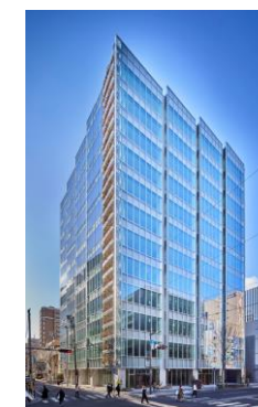
▲ T-PLUS Sendai (Completed in January 2024)
