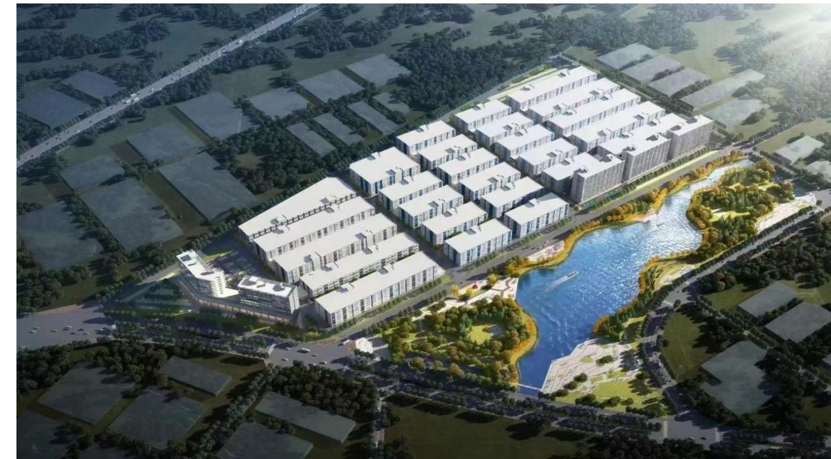
Mar 2023 Shunde Daliang new factory completed
