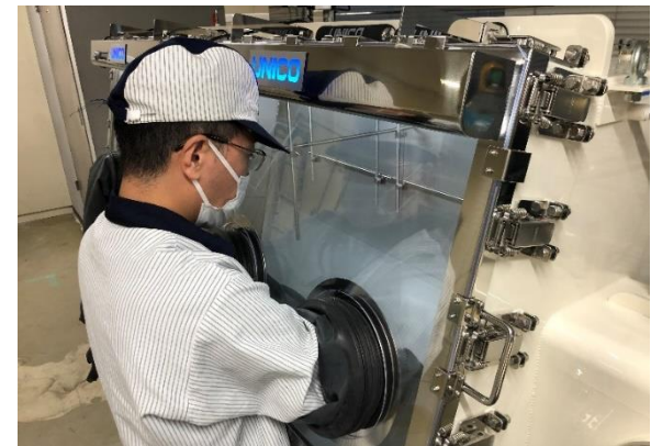
Glovebox for dismantling cells
