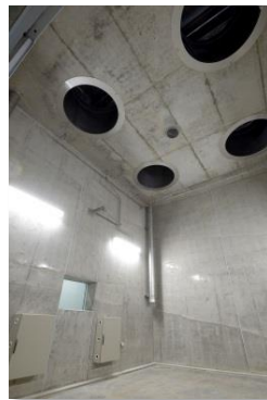
No. 2 Safety Test Room
