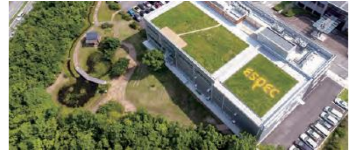
Rooftop green space using native species
