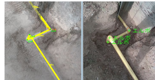
Technology to automatically create pipe construction drawings using 3D photography
