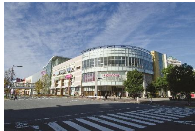
AEON MALL Chiba-Newtown (The shopping mall building and The cinema and sports building)
