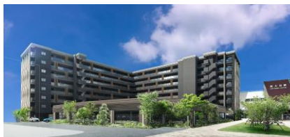
Le JADE Shin-Omura Station Front (first condominium project in Nagasaki Prefecture; multipurpose development project in front of the station)
