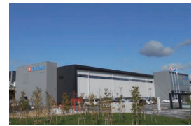
Shiga Ryuo Plant
