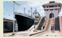
Electric towing locomotive for the Panama Canal
