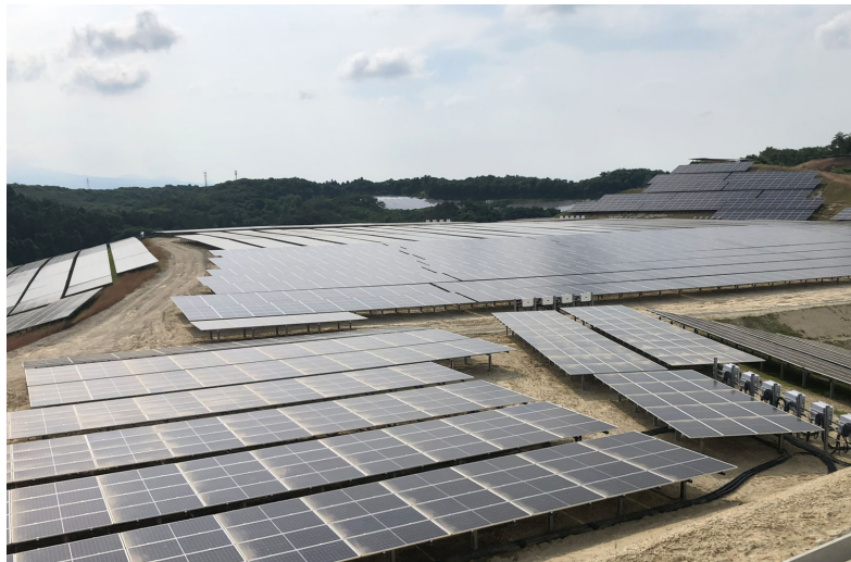
[Taiwa Town Solar Power Plant]
