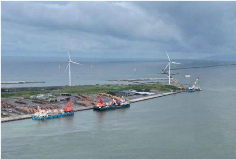
Offshore wind power generation business
