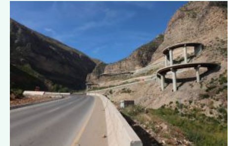
Pakistan – N-70 East-West Road Improvement Project
