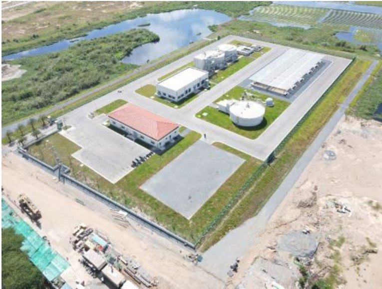
Completed sewage treatment plant (Nov. 30, 2023)
