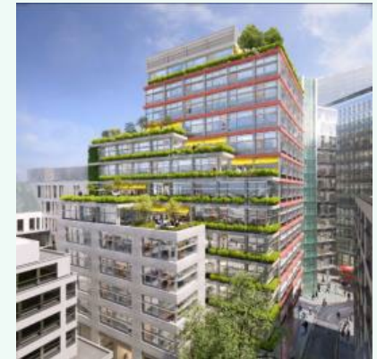
Pioneered the trial of Materials Passports* within the development of the "Edenica" commercial building.
